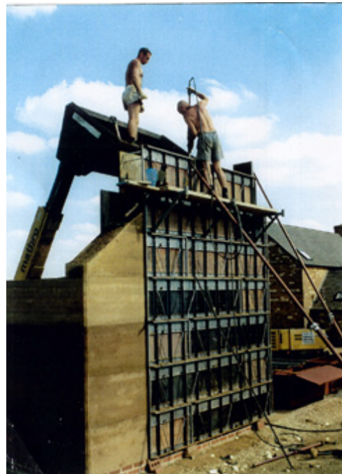
Figure 6.2: Modern Australian Formwork (Bill Swaney)
