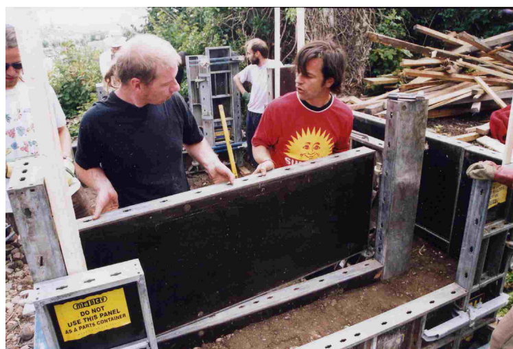
Figure 6.1: Modern concrete shuttering for rammed earth (photo: R.Keable)
