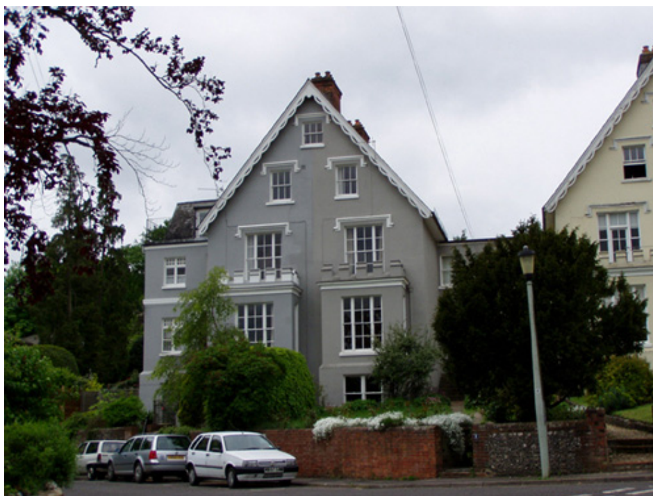
Figure 10.1: Five storey rammed chalk building in Winchester, Hampshire
